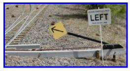
placed by the remote manual switches, but you will still find a few on the main line. To operate these switches, you simply move the arm to point it the direction you want to go. After you have moved your train through this type of switch you must realign the switch for the mainline.
