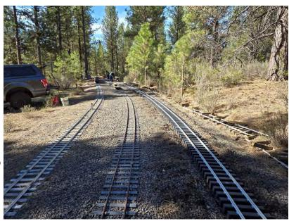
The last section of old wood ties were replaced with new aluminum on plastic ties, so the secondary main has now been upgraded the entire length of the main yard. Thanks go to Kim Beard, Kirk Devine, Jim Pendley and Chris Holland.
